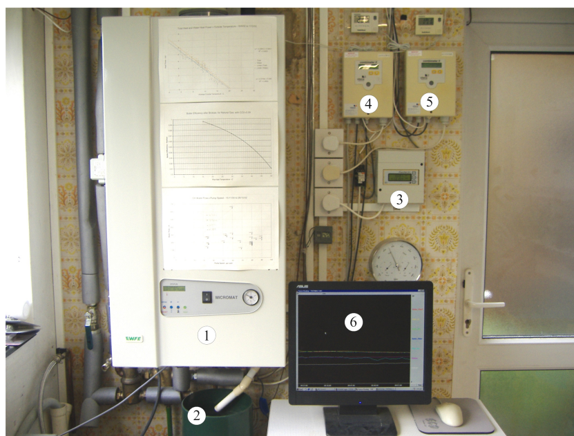
Fig. 2: 1 Boiler, 2 Rain Gauge, 3 Electricity sub-meter, 4 Heat Meter-Boiler, 5 Heat Meter-DHW, 6 Screen of Data Logger PC.
