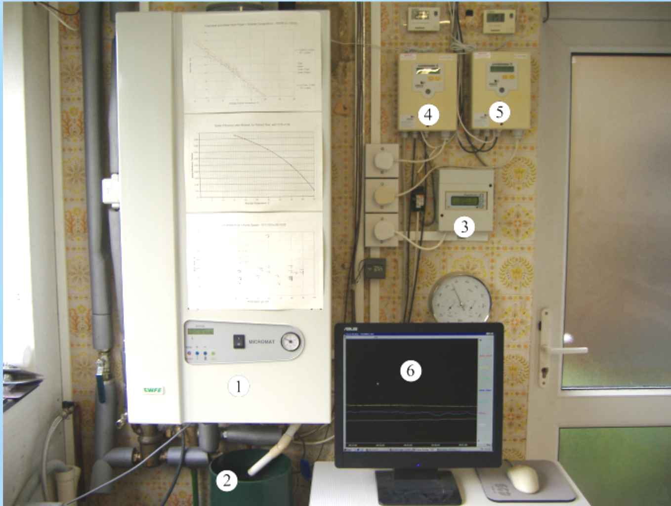
1 Boiler, 2 Rain Gauge, 3 Electricity sub-meter, 4 Heat Meter-Boiler, 5 Heat Meter-DHW, 6 Screen of Data Logger PC.
